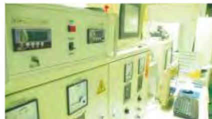
風洞實驗室 LAB OF TESTING FANS
